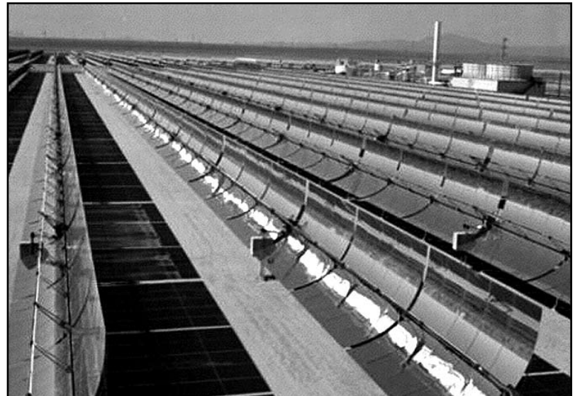
This CSP plant near Barstow, CA has been providing enough clean power for several hundred thousand homes since the 1980s. (Photo by Department of Energy)
